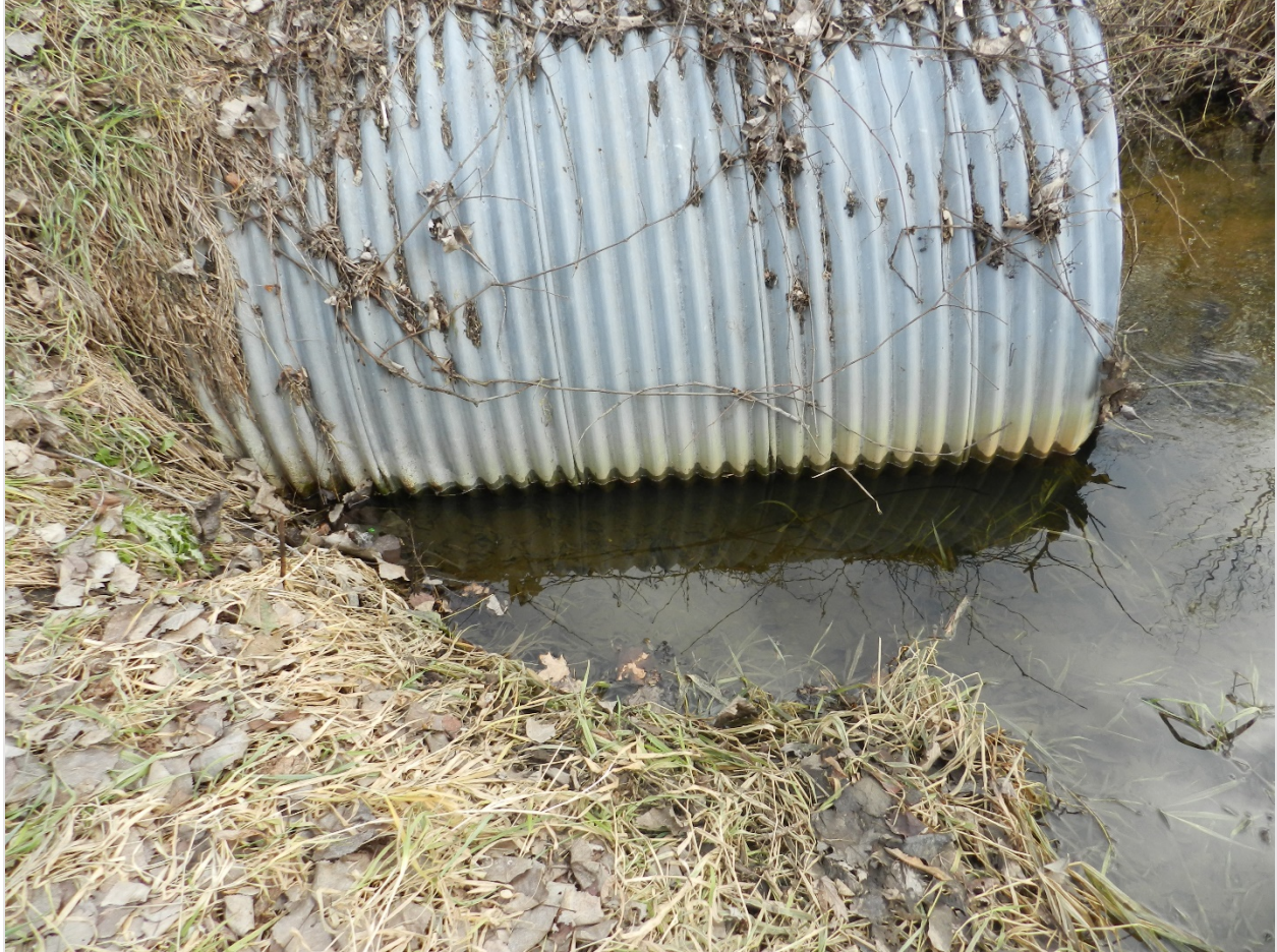
Figure 3.18 Upstream ponding from an undersized and perched culvert, Howard Drain culvert at Tyrrell Road – Howard Drain sub-watershed, Shiawassee County, Site 23.
