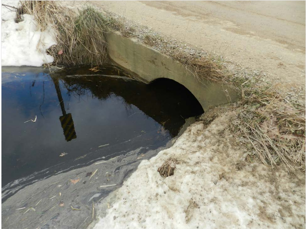
Figure 3.20 Road gravel eroding directly into waterway at unknown stream crossing at Winegar Road - Leisure Lakes sub-watershed, Shiawassee County, Site 27.
